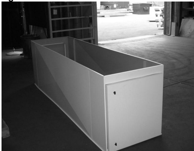
Figure 6: Fully assembled CRAC Extension on floor
